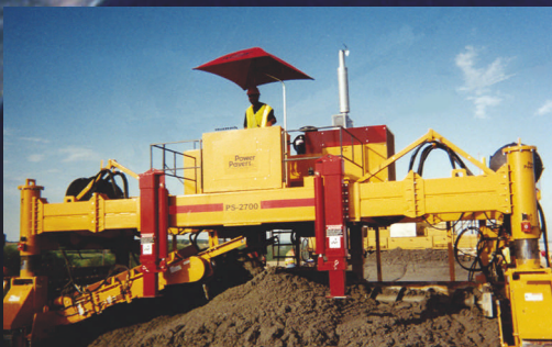
Power Paver PS 2700 Places and spreads concrete
